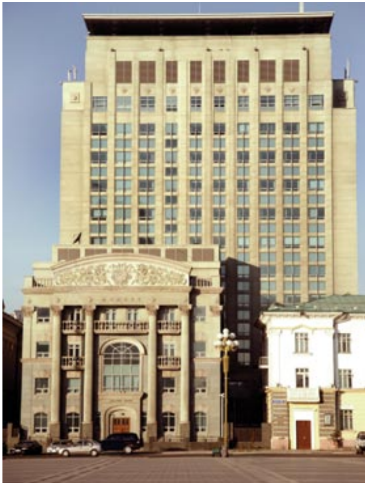
Golomt Bank Head Office (foreground) and Bodi Tower (background)
